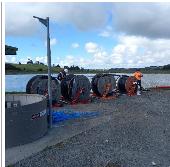
Cables ready to be pulled and load scales with remote display
