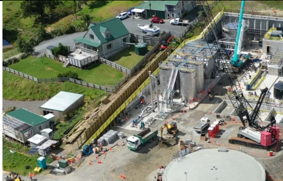
Timber Retaining wall installed
