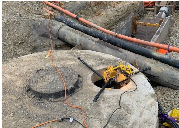
Laser scanning a site manhole without confined space entry.
