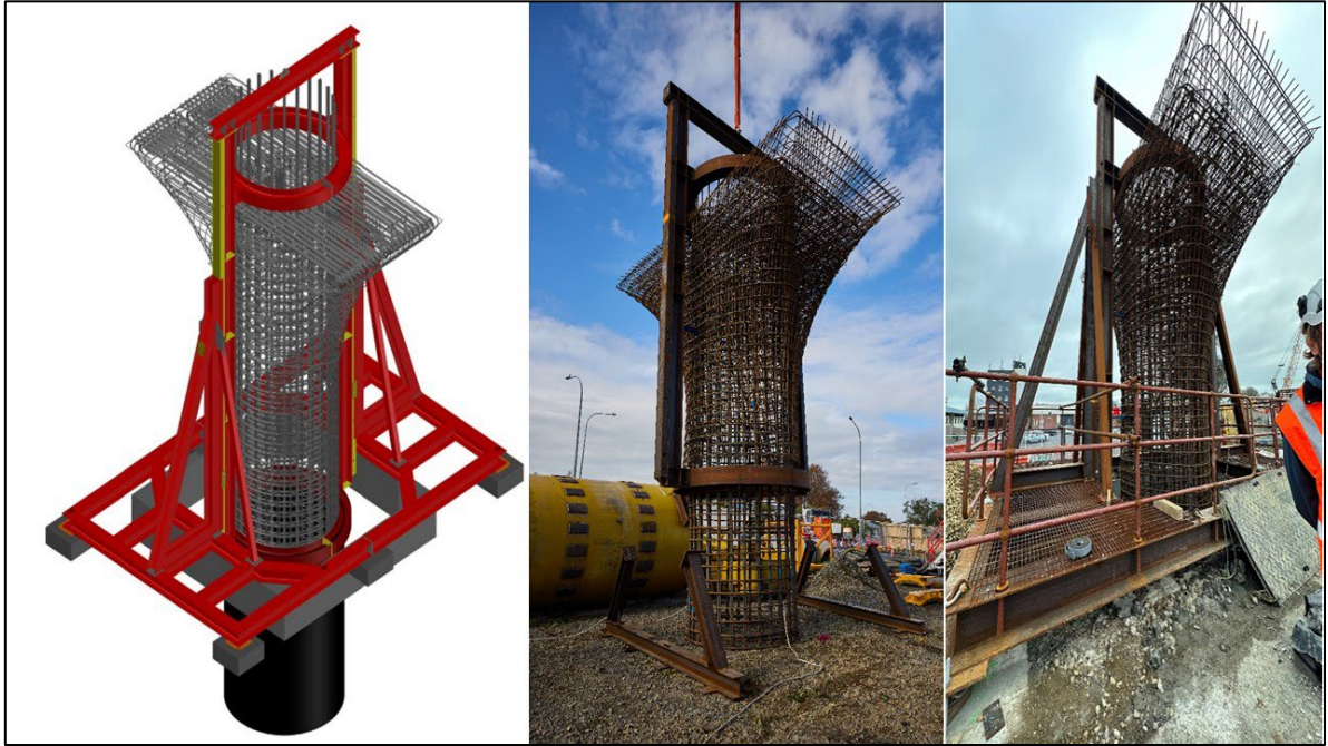
The flares lifted into place on site at EBA.
