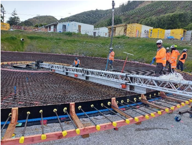
The unique vibrating screed in operation
