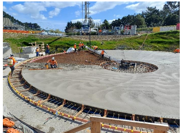
The unique vibrating screed in operation
